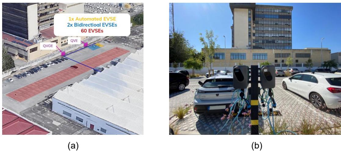
Figure 17– Aerial view of the parking lot in EDP campus (a) and existing chargers (b)
