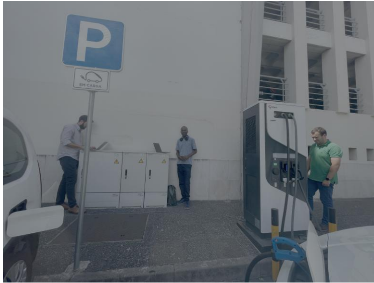
Figure 10 – Works being carried out during the commissioning of the EEM/EMACOM Fast Chargers.
