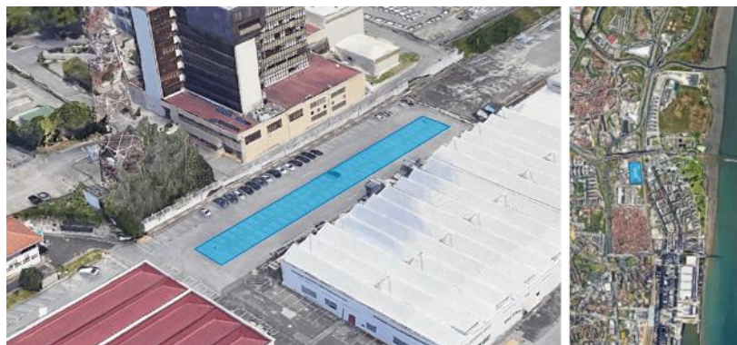
Figure 5 – Parking lot infrastructure in EDP installations.
